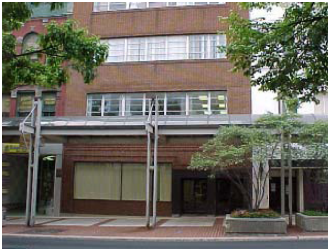
Allentown Community Corrections Center
